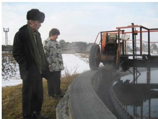
Grant funds were used to install ridged overflow edges made of organic glass
