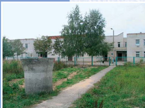
The water, heating and lighting systems were modernized in the building of Kindergarten #147 in Gorbatovka Settlement
