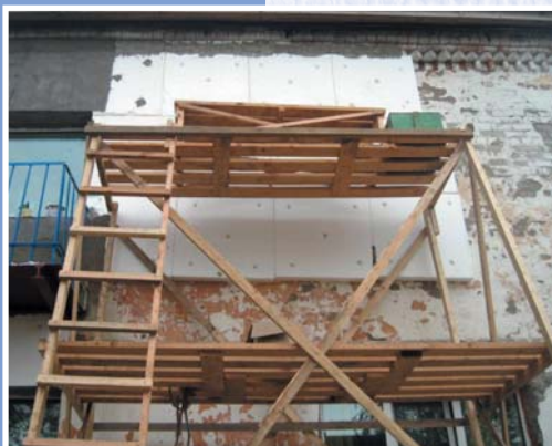
A residential building in the Family Hearth Village was winterized with the use of new heat insulating materials
