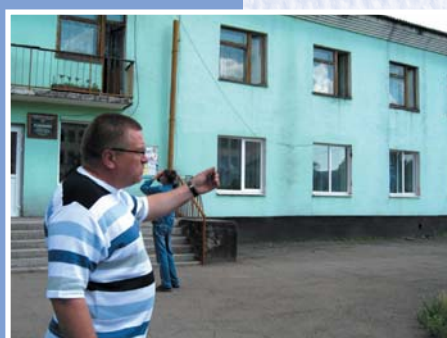
Head doctor of Svirsk Hospital, Vasily Tumin, points to the new windows and doors installed under the project in the children's and emergency departments of the hospital
